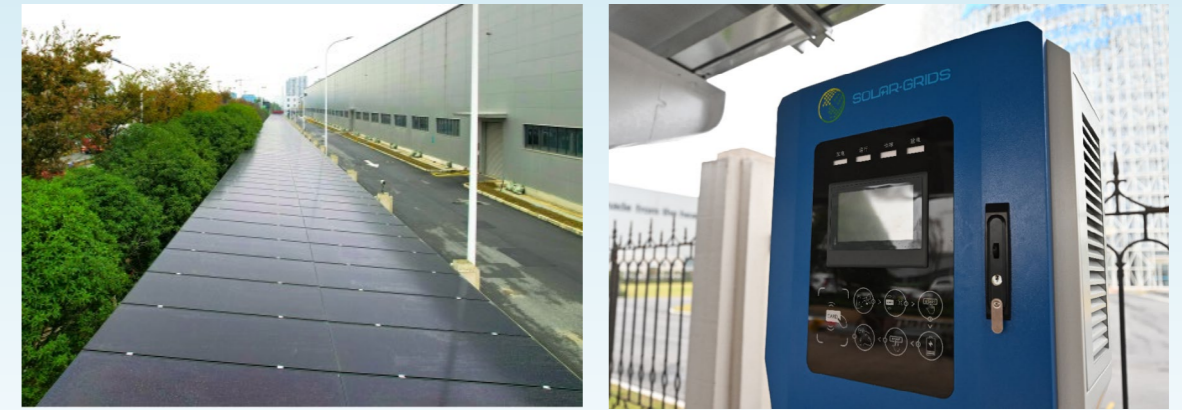
PV Car Parking Shed
