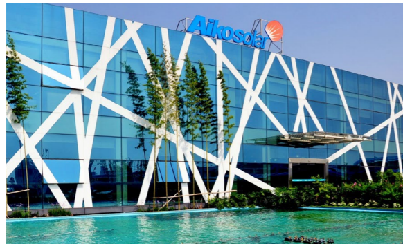
Foshan Base of Aiko Solar
