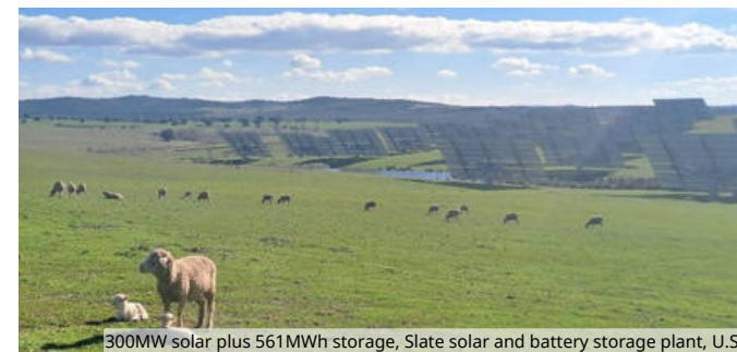
300MW solar plus 561MWh storage, Slate solar and battery storage plant, U.S.
