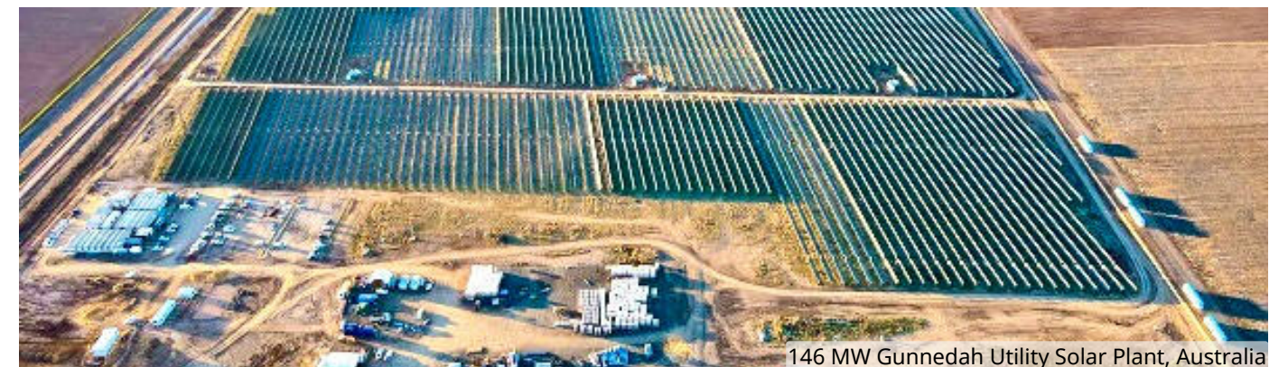
146 MW Gunnedah Utility Solar Plant, Australia
